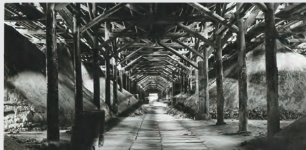
Calcium superphosphate warehouse
