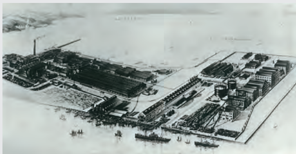
View of entire works after the first-phase ammonia plant completion
