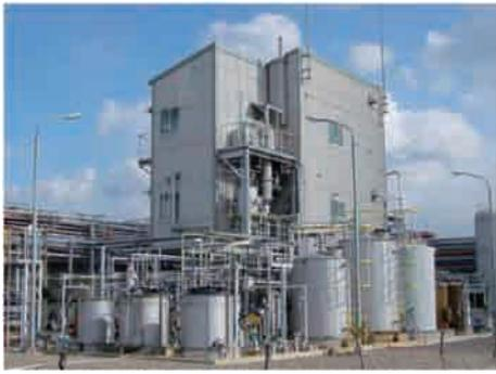
**Fig. 12** HCl oxidation demonstration pilot plant<sup>12)</sup>
