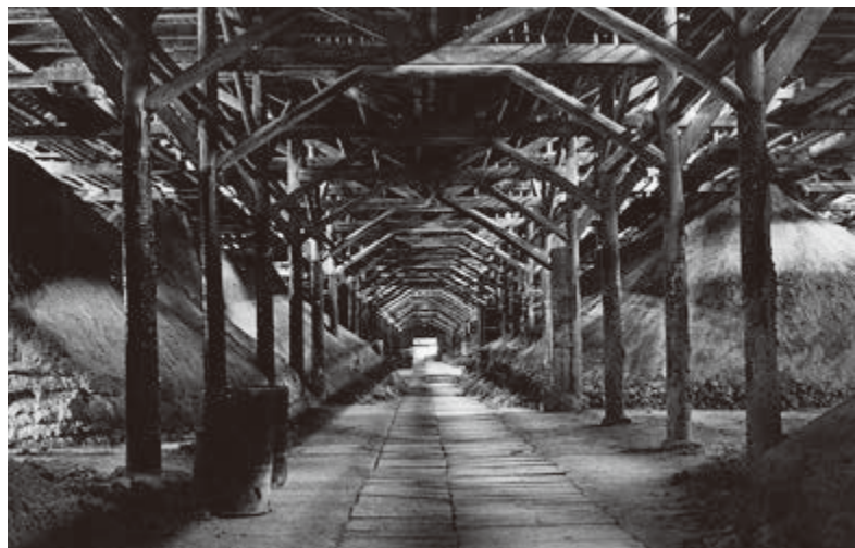
Calcium superphosphate warehouse
