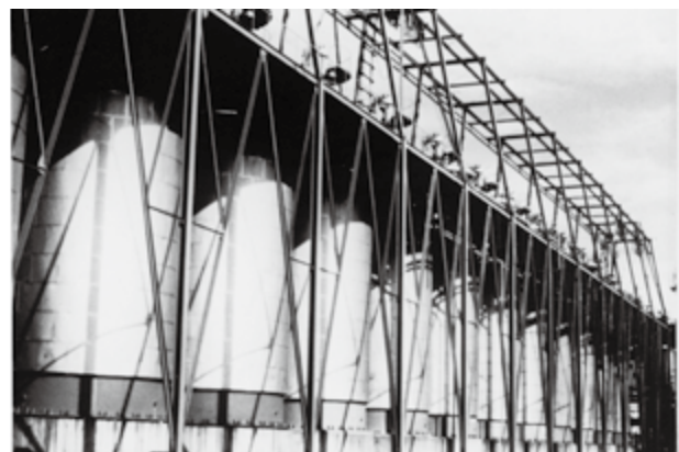
Alumina deposition tanks (Ehime)
