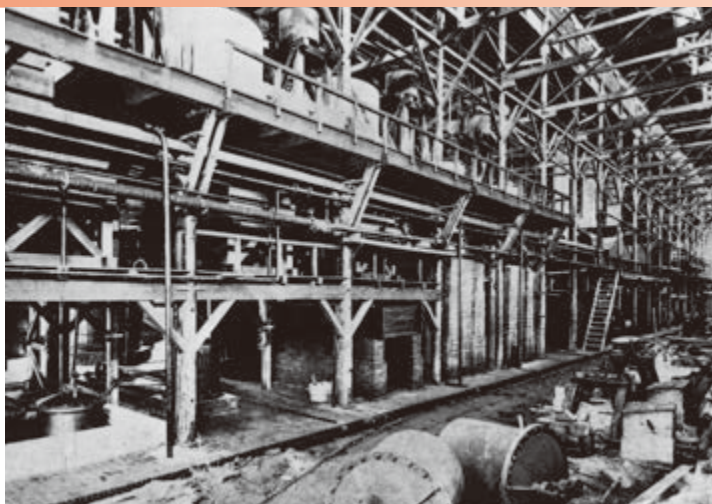
Interior of dyestuffs plant (Kasugade, Osaka)
