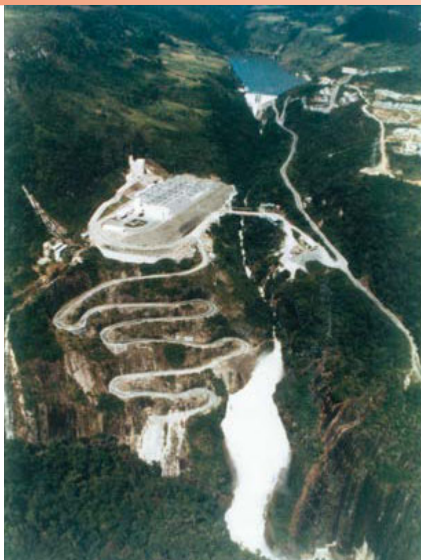
Sigura-gura Dam power generator, P.T. Indonesia Asahan Aluminium
