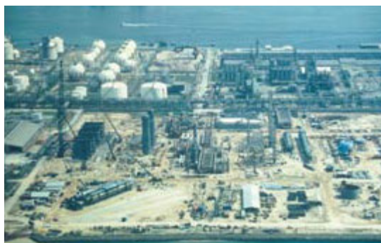
Construction site of PCS second phase ethylene facilities (Singapore)
