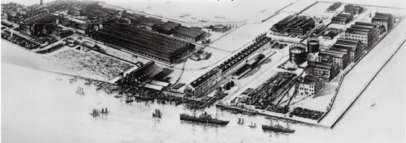
View of entire works after the first-phase ammonia plant completion (the ammonia plant is on the right)
