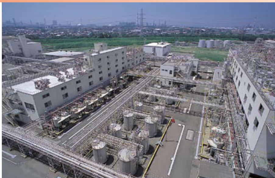
Plant for Meropen active ingredients (Oita)
