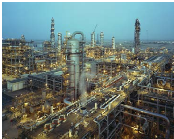
Rabigh Refining and Petrochemical Company complex
