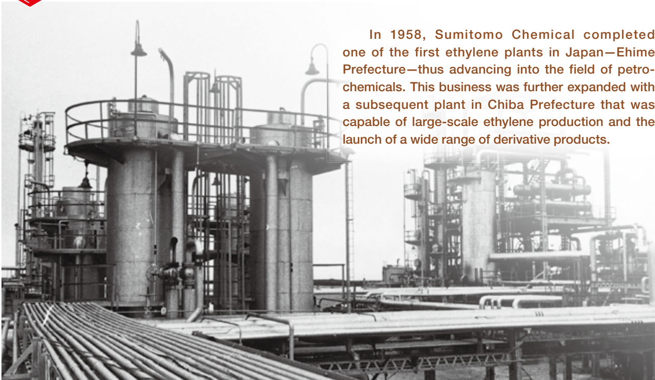
Ethylene plant (Ehime)
