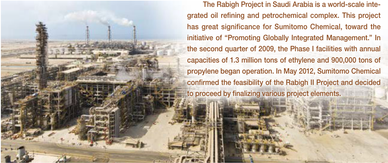
Rabigh Refining and Petrochemical Company complex
