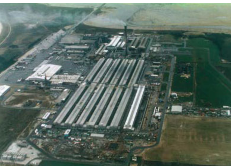
New Zealand Aluminium Smelters (NZAS) plant
