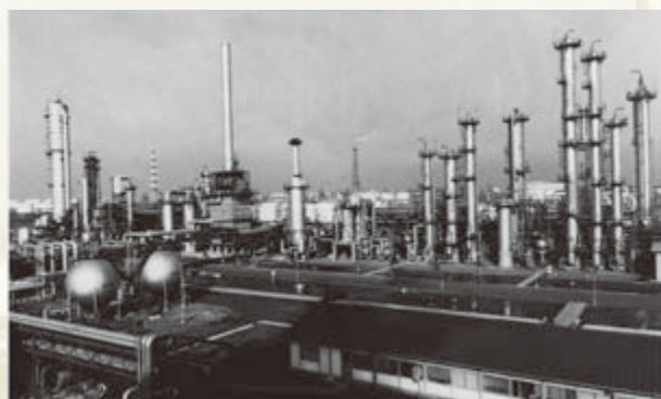
BTX plant and styrene monomer plant (Chiba)
