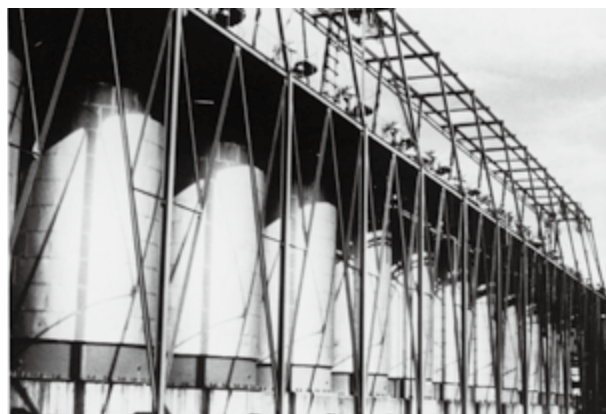
Alumina deposition tanks (Ehime)
