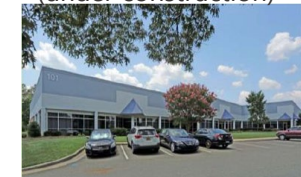
Sumitomo Pharma US cell production facilities
