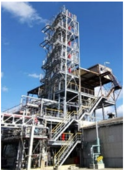
4 Chemical recycling demonstration facility
