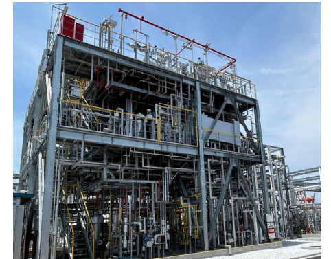
ETEP pilot plant exterior
