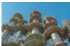
MMA plant in Singapore
