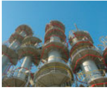
MMA plant in Singapore
