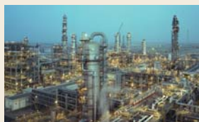
Rabigh Refining and Petrochemical company complex
