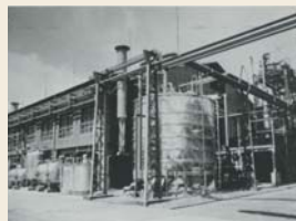
Pynamin Plant (Torishima, Osaka)
