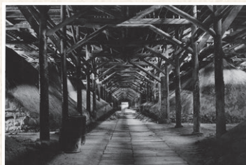
A 160-meter-long warehouse for calcium superphosphate
