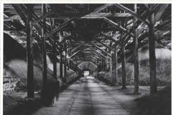
A 160-meter-long warehouse for calcium superphosphate
