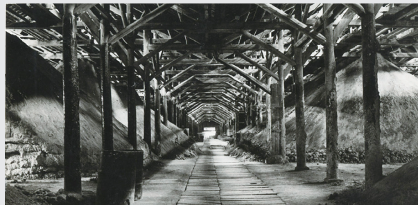
Calcium superphosphate warehouse
