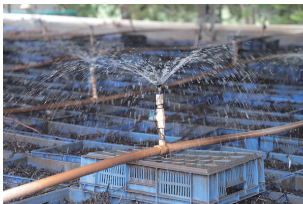
Treatment using earthworm farming technology instead of the common activated sludge method to suit the characteristics of household wastewater, which contains relatively high levels of nutrients
