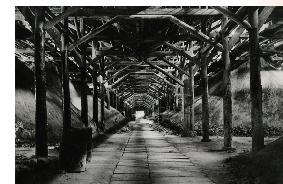
Calcium superphosphate warehouse
