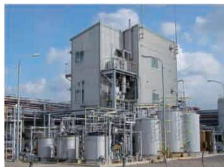
**Fig. 12** HCl oxidation demonstration pilot plant<sup>12)</sup>
