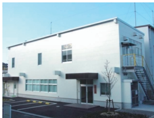
Fig. 5 The Experiential FE (Fire & Explosion) Training Center
