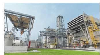
Niihama North Gas-Fired Power Plant
