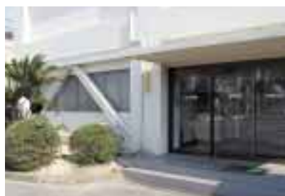
Ehime Works office reinforced with earthquake-resistant steel girders
