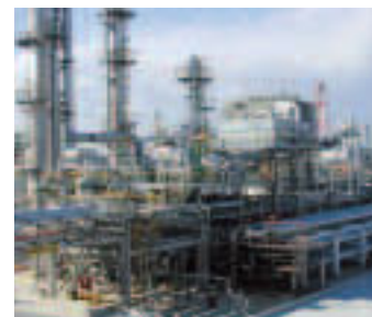
Nihon Oxirane's facilities for manufacturing propylene glycol
