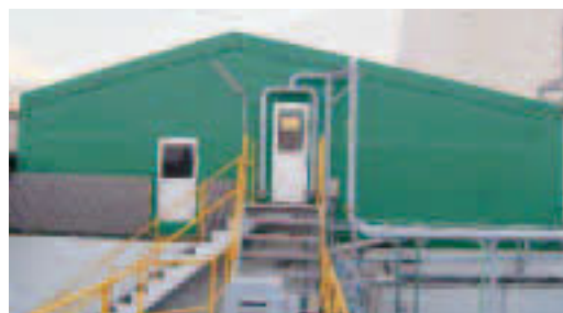
Tent containing aeration tanks
