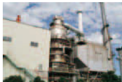
Fluidized-bed incinerator for treating wastewater and other material
