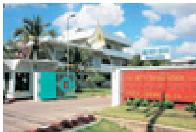
Bara Chemical's plant in the Bangpoo Industrial Estate, Samut Prakan, Thailand
