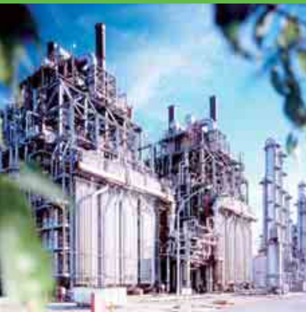
Sumitomo Chemical's major petrochemical manufacturing plants have been proven to be among the world's most energy-efficient through surveys conducted by the IEA and other organizations. This photo shows the ethylene plant (naphtha cracker) at the Chiba Works.
