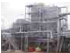
Main boiler with a feed-water preheater (top left)
