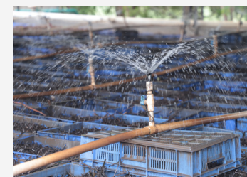
Water Treatment at the Bhavnagar Plant
