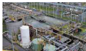
Activated sludge treatment facility
