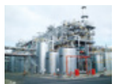
Vapor-phase caprolactam process equipment
