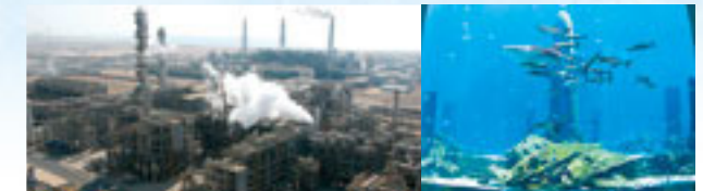
Petro Rabigh integrated oil refining and petrochemical complex (Saudi Arabia)
