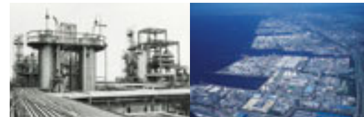
Ethylene plant (Ohe Works)
