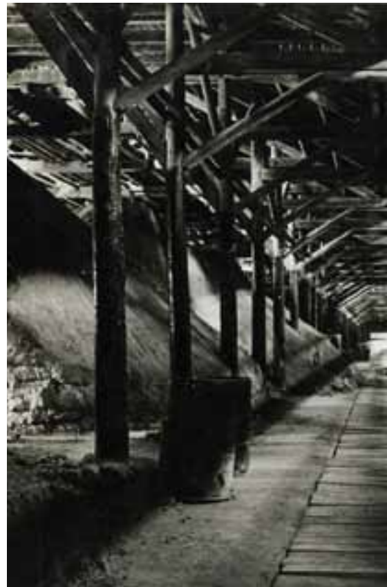
Warehouse of the fertilizer plant
