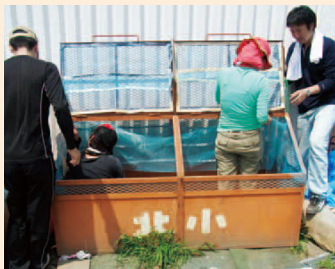
Installing a garbage collection point in a temporary housing area with an insecticidal net
