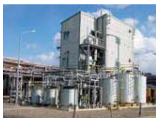
Hydrochloric acid oxidation process equipment
