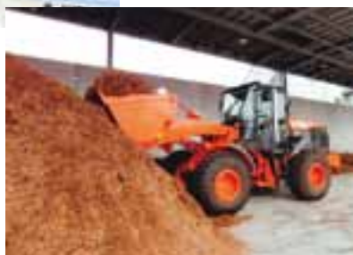
Transporting the crushed logging residues (Niihama-Nishi thermal power plant)
