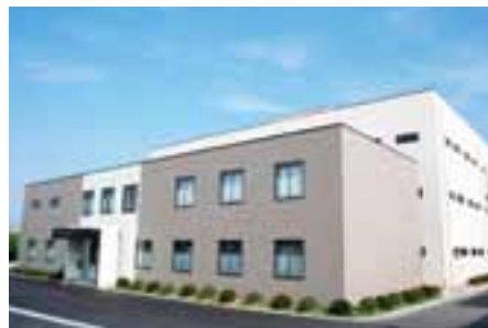
Sumika Chemical Analysis Service's Ehime Laboratory
