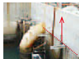
The height was increased in the seawater intake pump area
