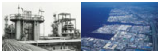
Ethylene plant (Ohe Works)
