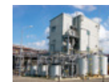
Hydrochloric acid oxidation process equipment
