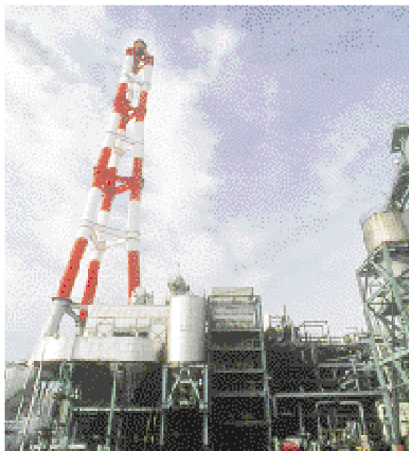
Proprietary technology used for denitrification
