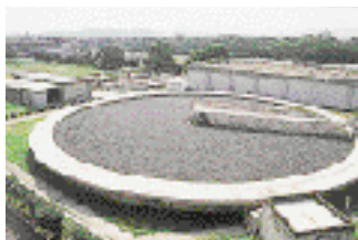
Wastewater treatment plant
