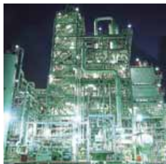
Gas-phase polypropylene manufacturing facility
