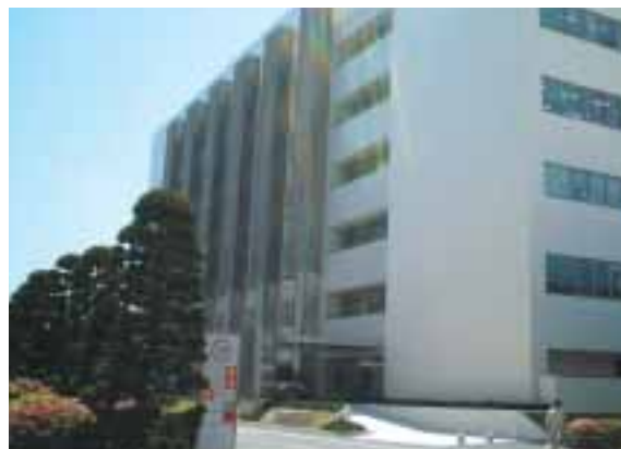
Organic Synthesis Research Laboratory and Process & Production Technology Center (on the site of the Osaka Works)
