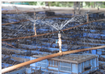
Water Treatment at the Bhavnagar Plant
