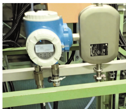
Fig. 18 Endress+Hauser, Proline Promass A 300, coriolis flow meter
