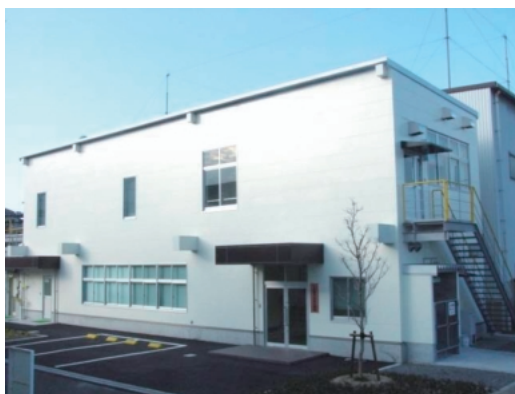
Fig. 5 The Experiential FE (Fire & Explosion) Training Center FE体感研修棟
